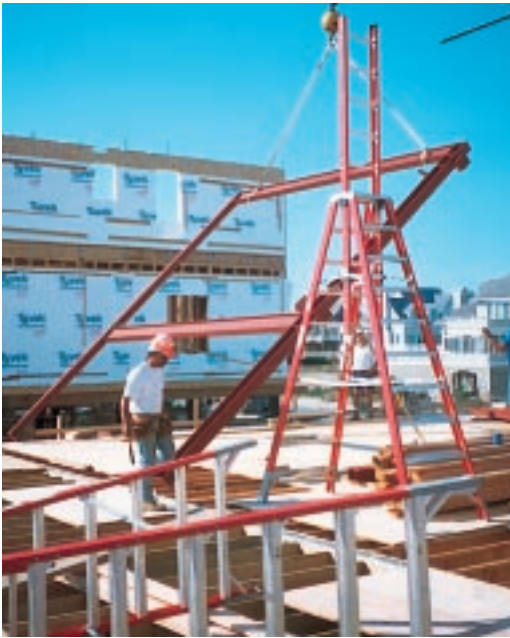
Figure 3. The author erected the moment frame in two main sections, then dropped connecting beams into place.
