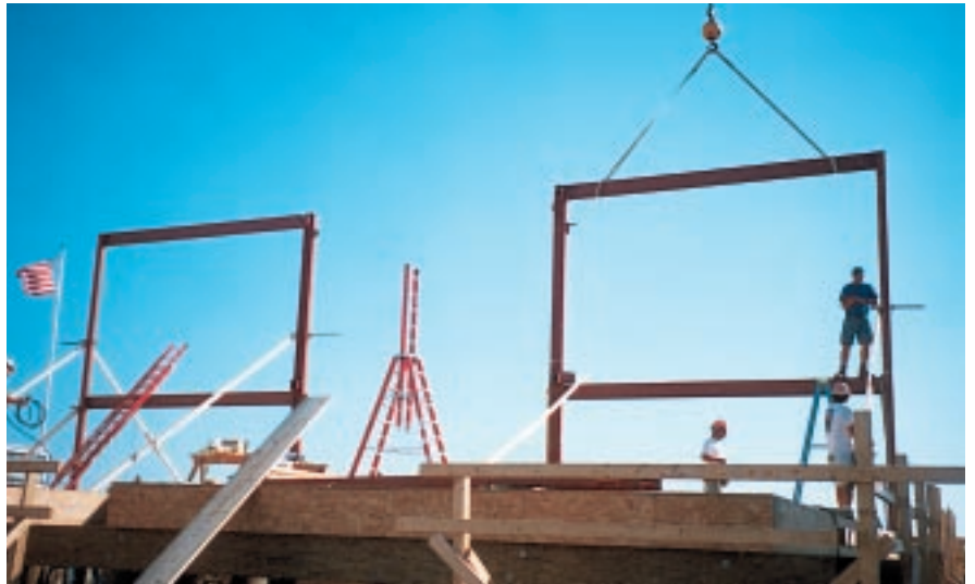
Figure 3. The author erected the moment frame in two main sections, then dropped connecting beams into place.
