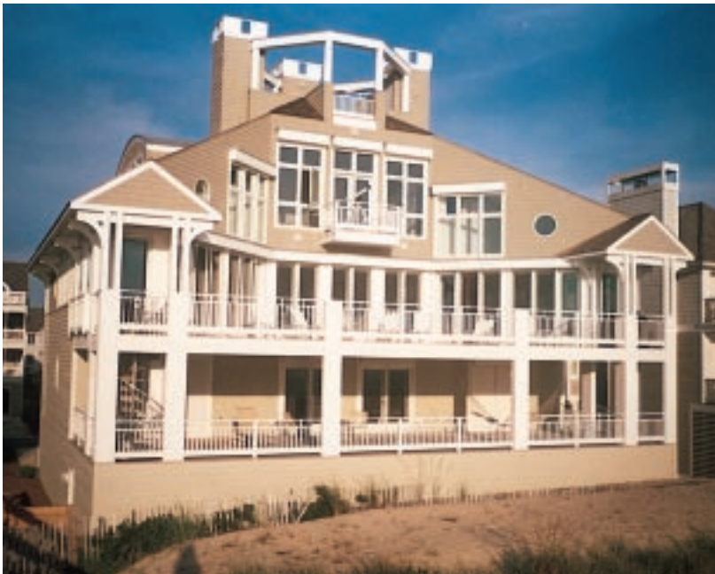
Figure 1. The expanse of windows walls in the east wall of this oceanfront home leaves no room for plywood shear walls (left). A structural steel moment frame embedded in the framing (right) handles large lateral wind loads.
