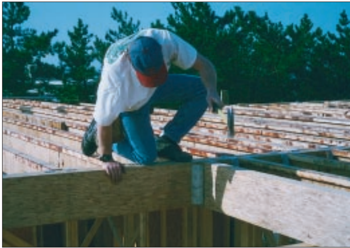
Unlike steel, Parallam integrates easily into a wood-frame structure, requiring only standard carpentry tools.
